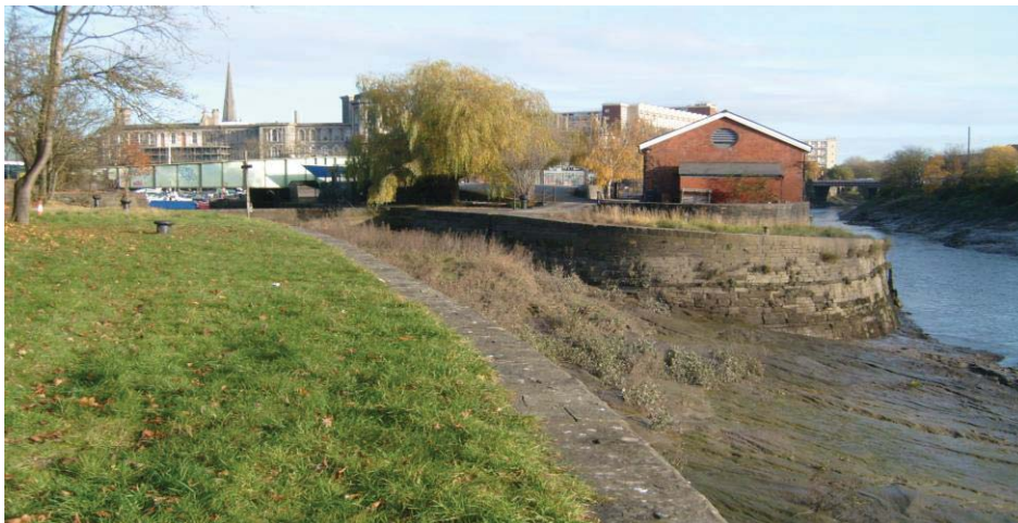
The blocked-up Bathurst Basin lock – a weak link in the City's defences
